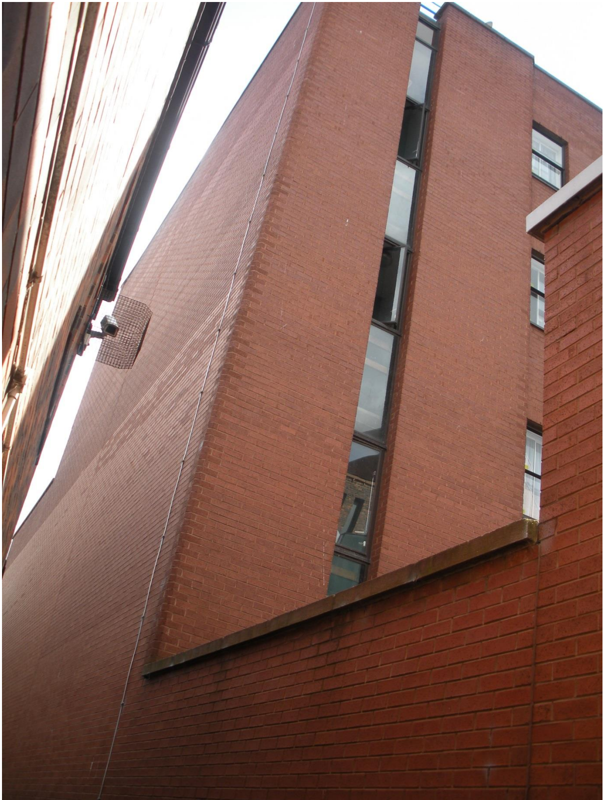
No.4. Looking up towards the hotel from the 'Courtyard' entrance.
